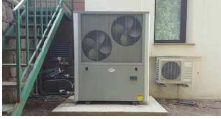
CEM ATAÇ EV ISITMA ve SOĞUTMA NEWTHERM AIRMINI AW08-8 kW + 7xFANCOIL
