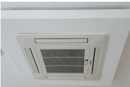
THE LIFECO-JUICE BAR-TÜRKBÜKÜ NEWTHERM KASET TİPİ FANCOİL
